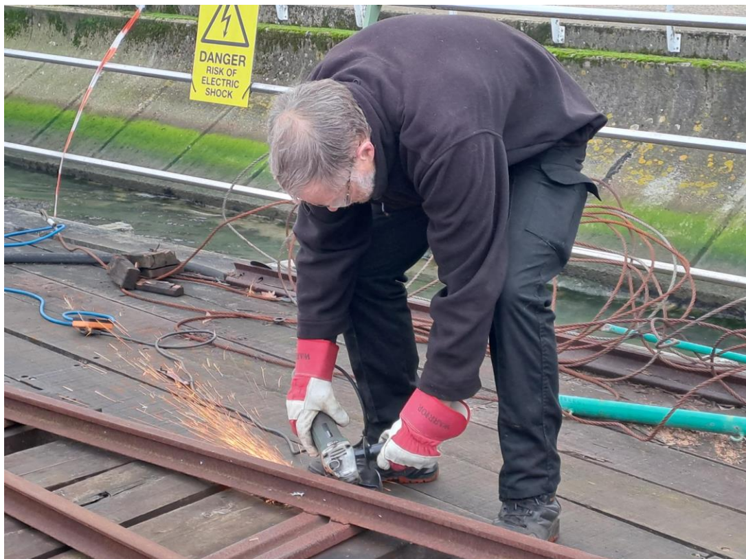
Below: Cutting old points prior to removal (Photo Alan Titheridge)
