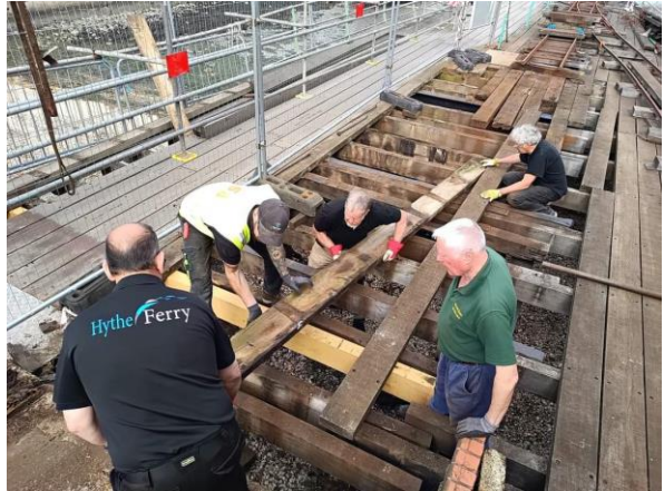
Above left: Jumble of beams, old and not so old revealed and Above right: First of new beams being slid into position, catching old beam (Photos John Greenwood)
