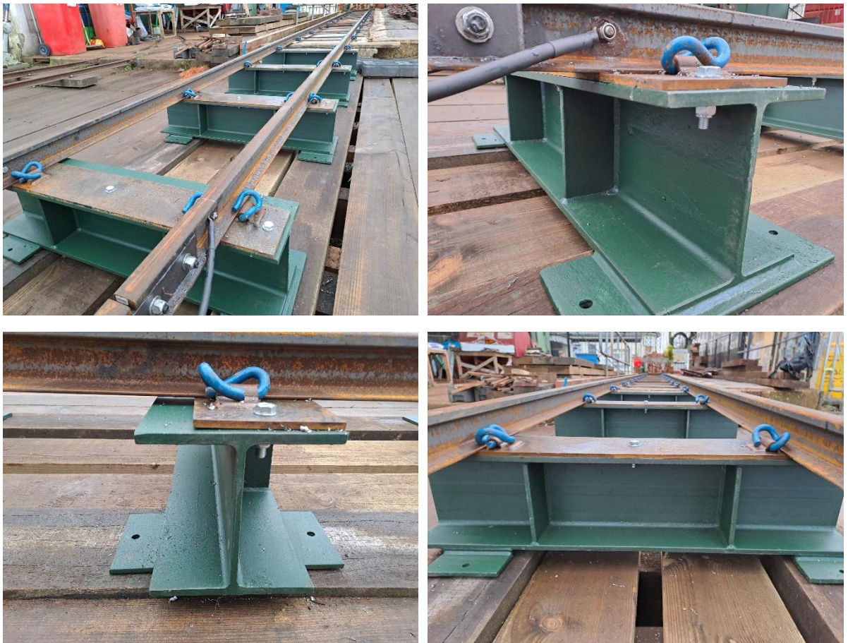
Above four images - Metal Sleeper Supports (unsecured) - Photos: Alan Titheridge
