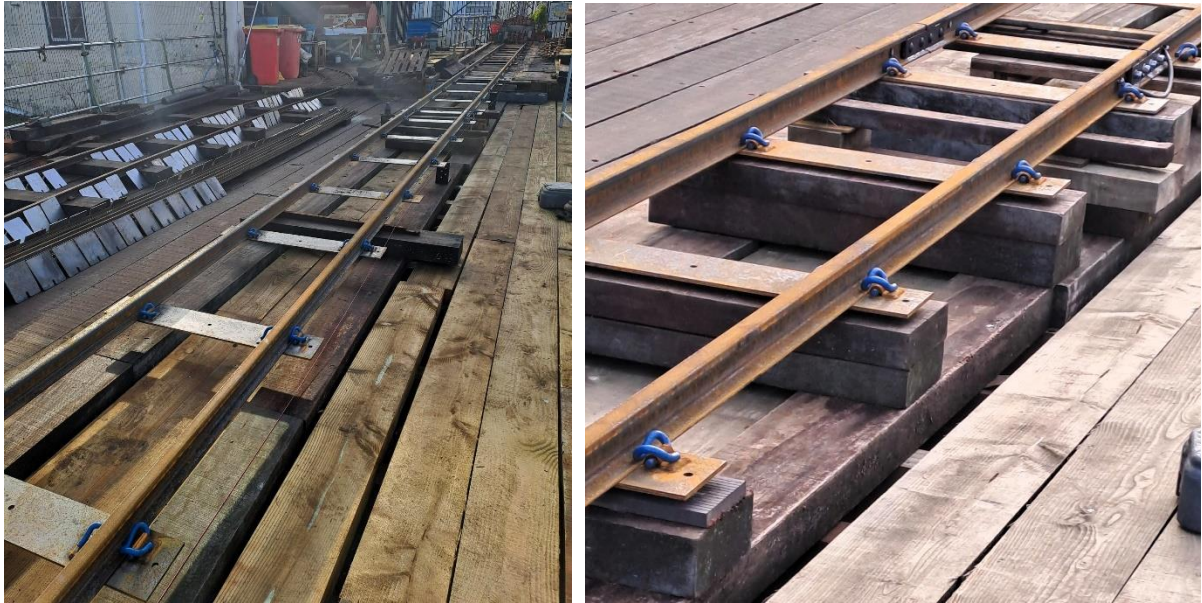
Above Left: Raised track prior to laying of wooden sleepers and Above Right: with wooden sleepers in place (unsecured) (Photos: Alan Titheridge)
