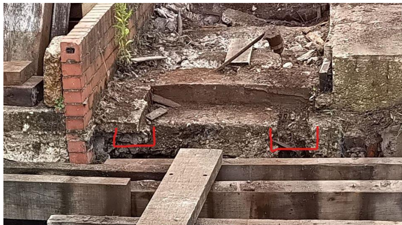
It appears the initial tracks were laid in 1922 without sleepers (John Greenwood)
