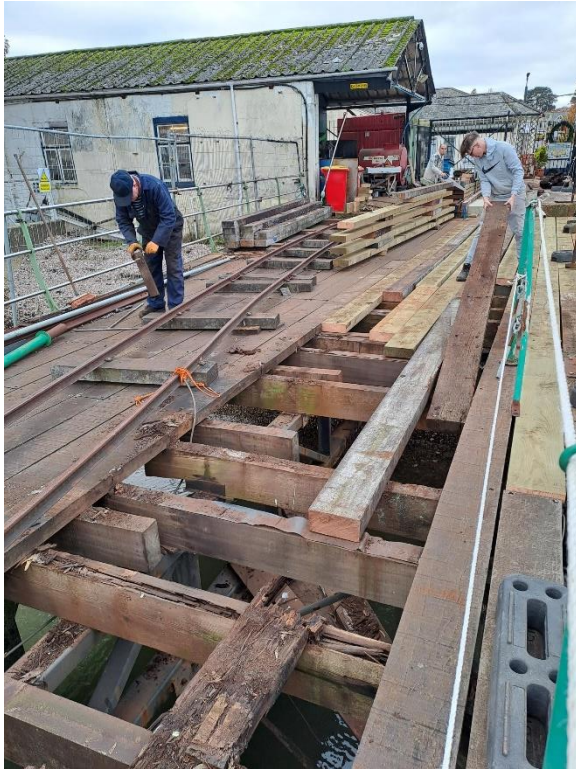
1Above: Positioning of new planks (Photos Alan Titheridge)
