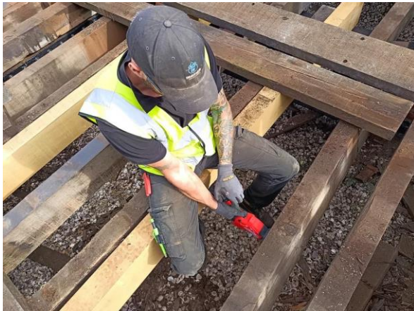
Above left: First new beams in position, removal of old beams that appear to have been ineffective for some time and Above right: Seven new beams in position (Photos: John Greenwood)
