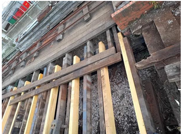
Above left: First new beams in position, removal of old beams that appear to have been ineffective for some time and Above right: Seven new beams in position (Photos: John Greenwood)
